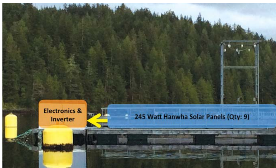
General layout of the 2.2 kW renewable energy system to power the SEATram at Kyuquot SEAFoods Ltd. This solar photo-voltaic system will provide clean energy throughout the year, reducing farm greenhouse gas (GHG) emissions and improving shellfish grading and harvesting operations. Photo: Stephen Cross (UVic)
