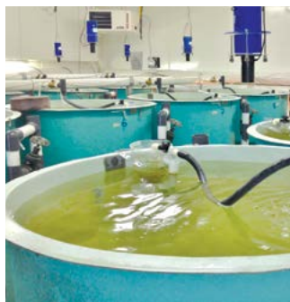
Conical rearing units with individual hatching jars and vibratory feeders hanging above. Photo: White Lake Fish Culture Station (OMNR)
