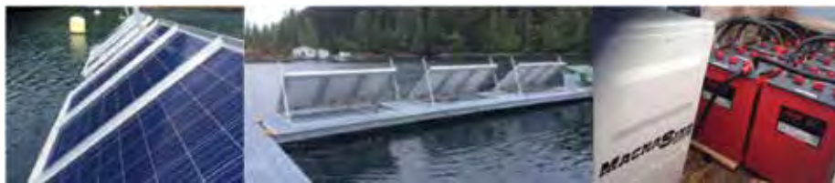
Installed renewable energy system components at Kyuquot SEAFoods Ltd. site: modular solar panels on dock (left and middle) with battery storage and power electronics in locker (right). Photo: Stephen Cross (UVic)
