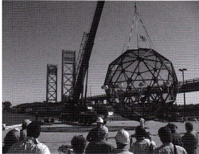
Figure 4 A 500-m 3 AquaPod™ fish pen being deployed at the Port Authority in Portsmouth, NH.
