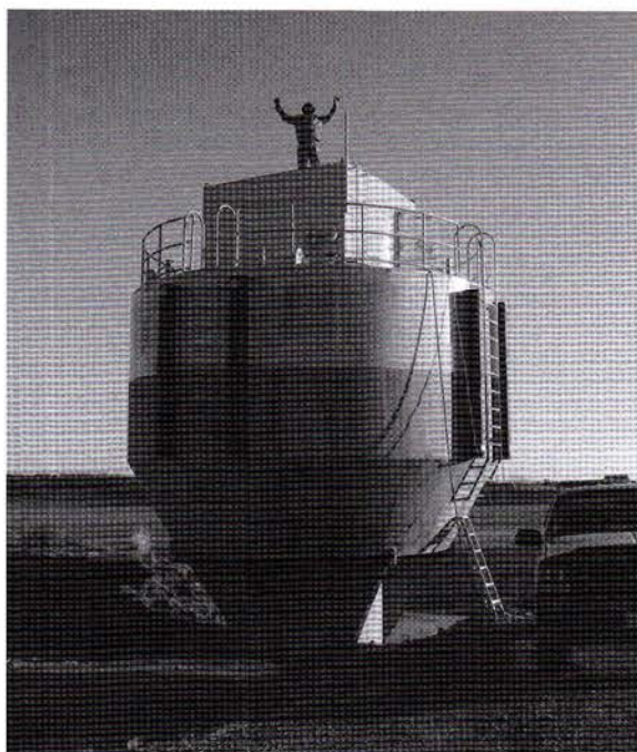
Figure 6 The 20-ton feed buoy under construction at AEG, Hillsborough, NB, Canada.
